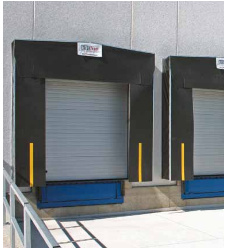
Lisbon Loading bays for logistic operations.
