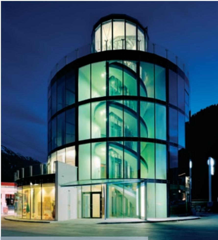
*A frameless, point-supported glass facade was created for the Bluetower in St. Johann with SCHOTT fire resistant glazing. The connection of the double-glazed elements with PYRAN® S was achieved using purpose-built steel sections, which were attached with stainless steel point fittings at each intermediate floor.*
