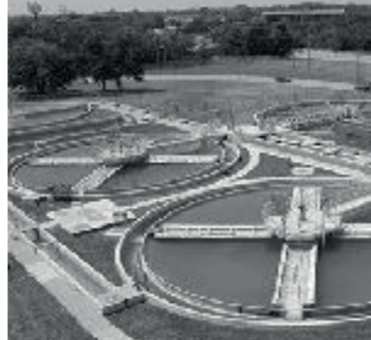
Water Treatment Center
