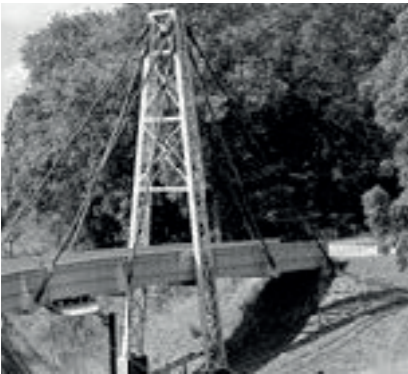
Bridge, Kolding Denmark
