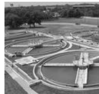
Water Treatment Center
